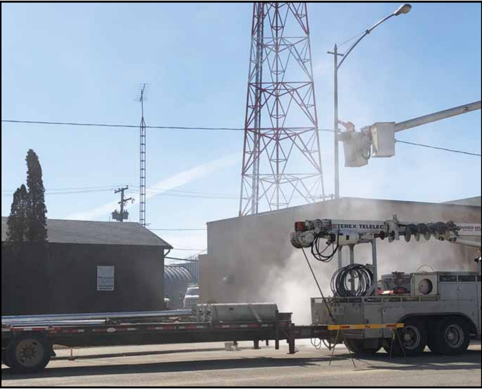
► After a wind storm toppled over a few streetlights last summer along Main Street in Watrous, crews were in Watrous last week swapping out a number of other standard streetlights along Main Street. Joel Cherry with SaskPower said a total of 19 standard streetlights were being replaced in town. The streetlight structures were encased in sidewalk concrete so crews were cutting out the concrete base and removing it before the replacements could take place. Weather permitting, SaskPower anticipated the work would be completed by the end of last week. photos by Daniel Bushman
