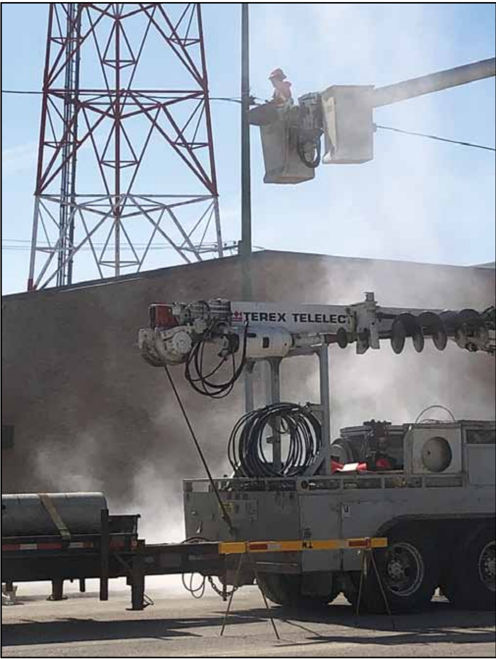
► After a wind storm toppled over a few streetlights last summer along Main Street in Watrous, crews were in Watrous last week swapping out a number of other standard streetlights along Main Street. Joel Cherry with SaskPower said a total of 19 standard streetlights were being replaced in town. The streetlight structures were encased in sidewalk concrete so crews were cutting out the concrete base and removing it before the replacements could take place. Weather permitting, SaskPower anticipated the work would be completed by the end of last week. photos by Daniel Bushman
