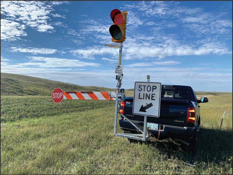
► Created by Watrous residents Kim and Donna Kreutzer, the Guardian Angel, a remote controlled automatic flagging assistance device is being tested in work zones in Saskatchewan. As part of a provincial pilot program, three sets of two of the
